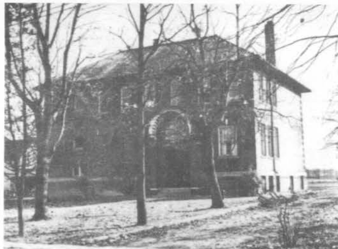
In 1929 an addition was built on to the east side of the school and separate entrances were created for boys and girls along with two new classrooms.
